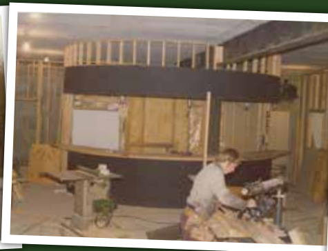
Construction of the main bar fall of '74
