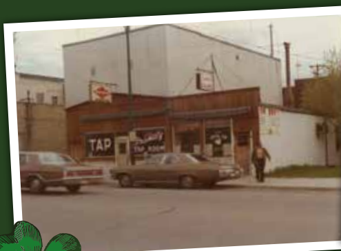
Friendly Tap, 310 Beltrami Ave June '74 prior to demolition
