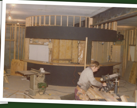
Construction of the main bar fall of '74
